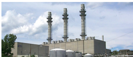
Pittsfield plant (Source: Maxim Power)
